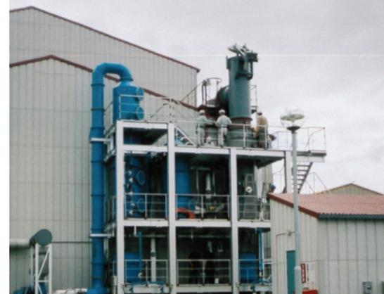
Flue gas treatment for precious metal recovery smelter, Japan
