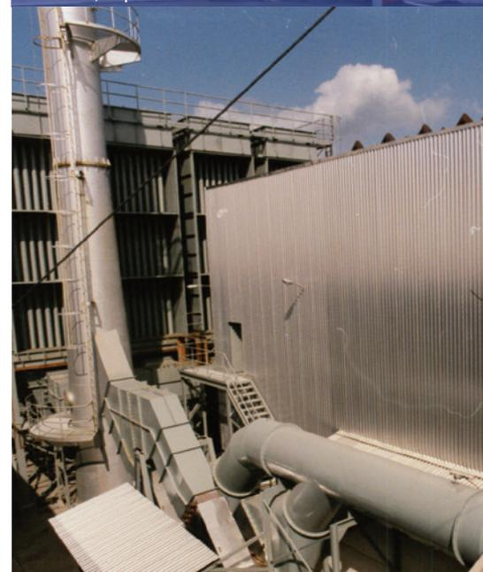
Zinc smelter reverberatory furnace flue gas treatment, Malaysia
