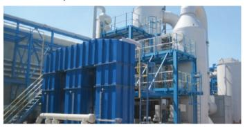
The high temperature of the gas meant that only a ceramic filter would be able to remove the majority of the entrained fibre content - protecting the downstream equipment from clogging.
