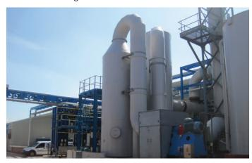
The materials of construction for the treatment plant had to be considered very carefully due to the highly corrosive (HCI) nature and temperature of the gas stream. The ceramic filter, the sub cooler and the RTO were constructed in Hastelloy C22, a high grade steel.
